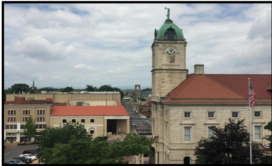
View of Courthouse Square from Axon AI's office
